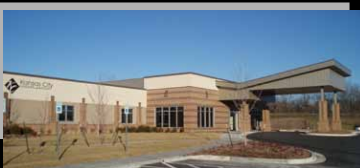
Green Hills Road & Hwy. 152 Kansas City, Missouri
